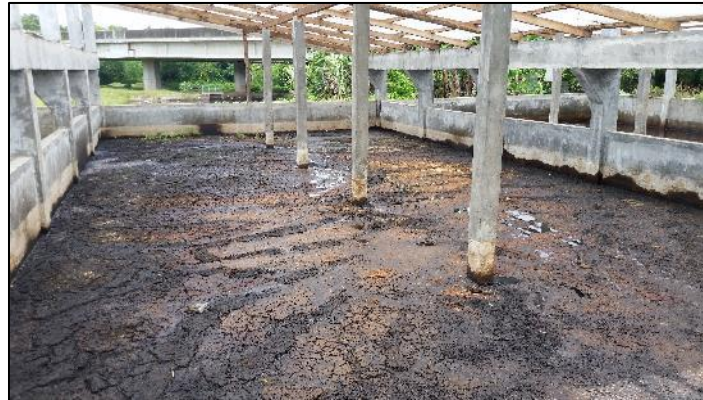
FOG on drying beds due to bypassing ABR
