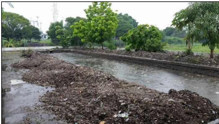
Bypassing initial grit removal due to lack of wash water
